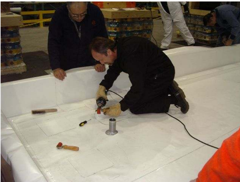
PVC Deck, Proper Welding Procedure for Repairs.
