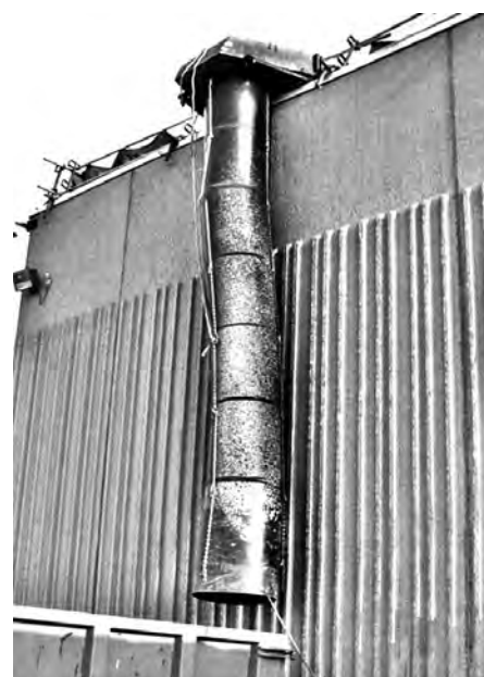
Use a Chute to Lower Garbage from Roof
