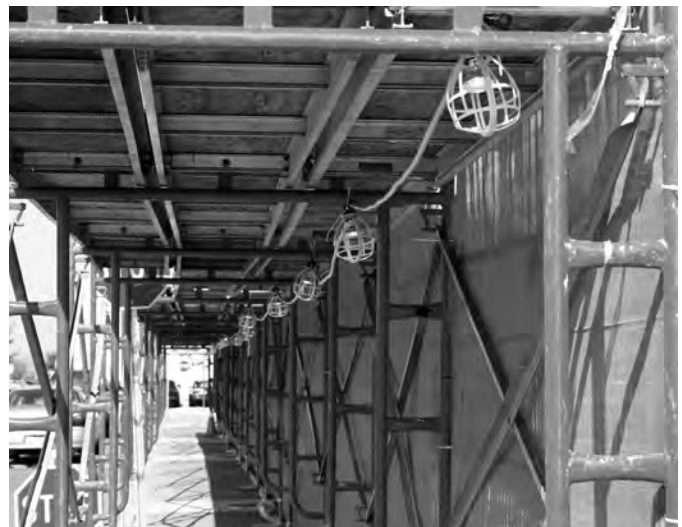
Temporary Lighting in Public Way Protection
