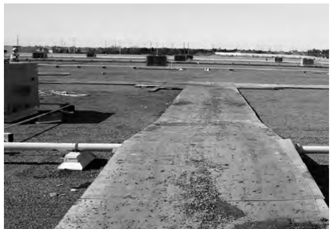
Be Careful When Installing Ramps over Gas Lines
