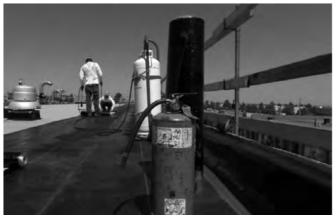
Have a Fire Extinguisher Available
