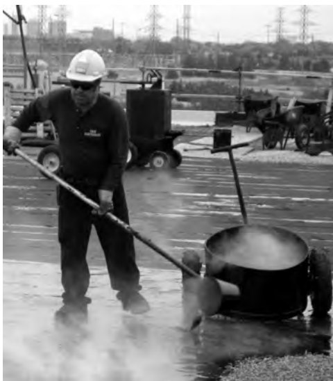
Cover Skin and Wear Gloves When Working with Asphalt
