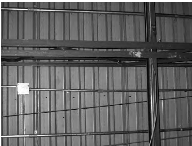
Electrical Conduit on Underside of Roof Deck
