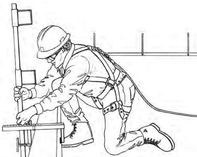
Fall Protection When Installing Guardrails
