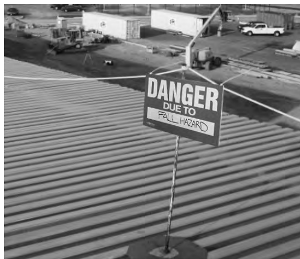
Warning Barrier with Danger Sign
