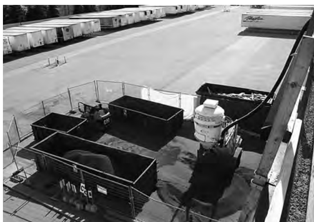
Vacuum Discharge Area
