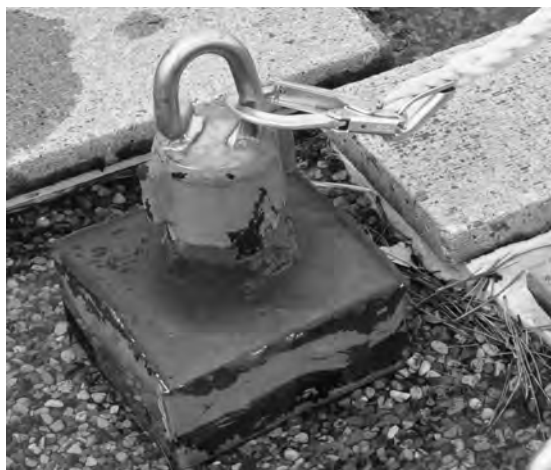
Roof Anchor (Designed Fixed Support)
