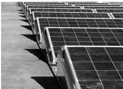
Ballasted PV system
