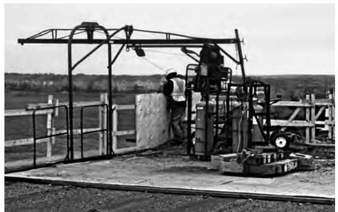
Typical Roof Hoist System
