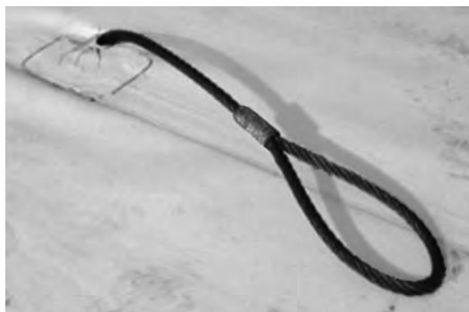
Temporary Anchor Fastened to Existing Structure
