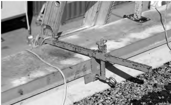
A Parapet Clamp Can Be Used to Secure Ladder
