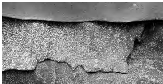
Check Old Roofing Materials Before Work Begins
