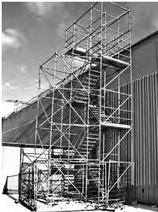
Scaffold Stair Tower
