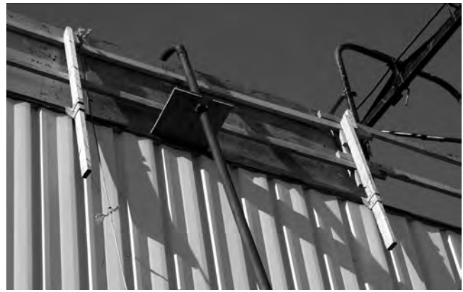
Asphalt Pipes at Roof Level
