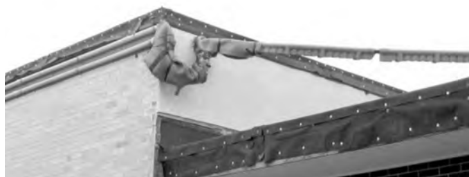
Powerline with Protective Insulation
