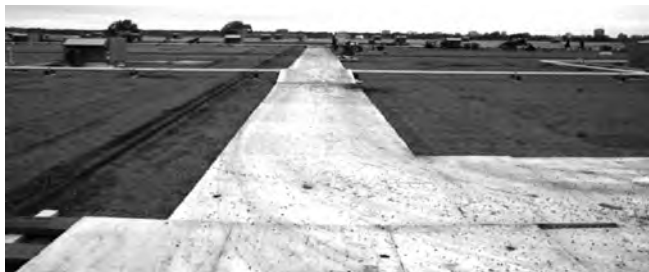
Use Plywood to Make Moving Materials Easier
