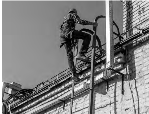
Fixed Access Ladders May Be in Poor Condition
