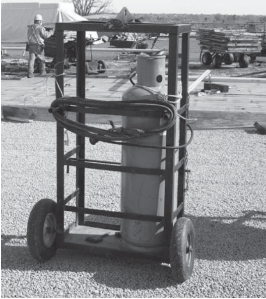
Propane tank, upright and secured on a cart
