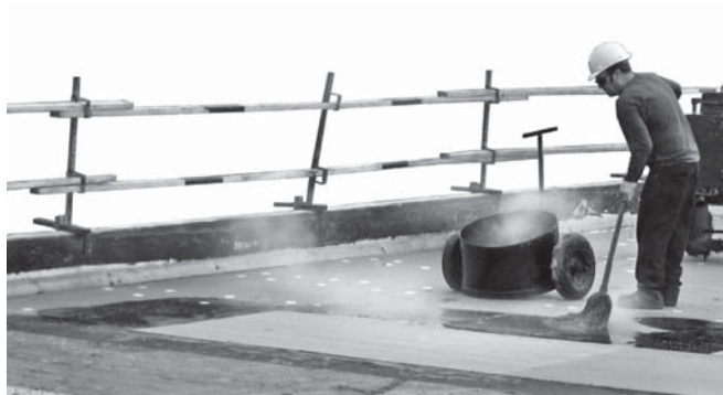
Guardrail system in place
