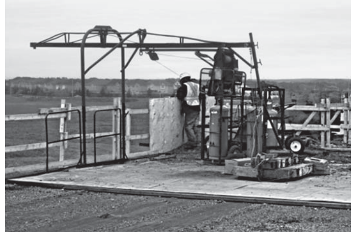
Typical roof hoist system
