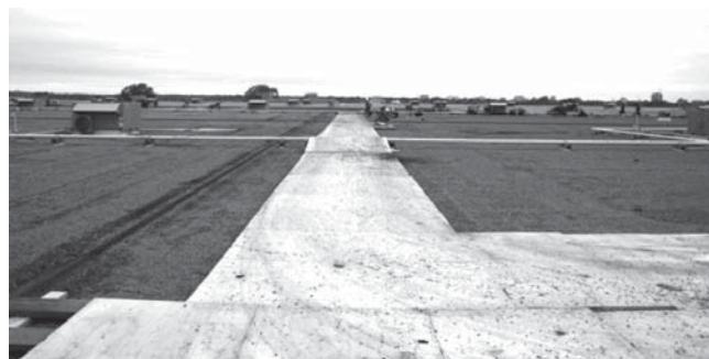
Plywood makes it easier to move materials
